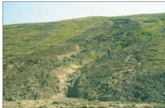
A landslide. Volcanic soils (Andosols) on slopes are very susceptible to disturbances such as clearing and overgrazing.
